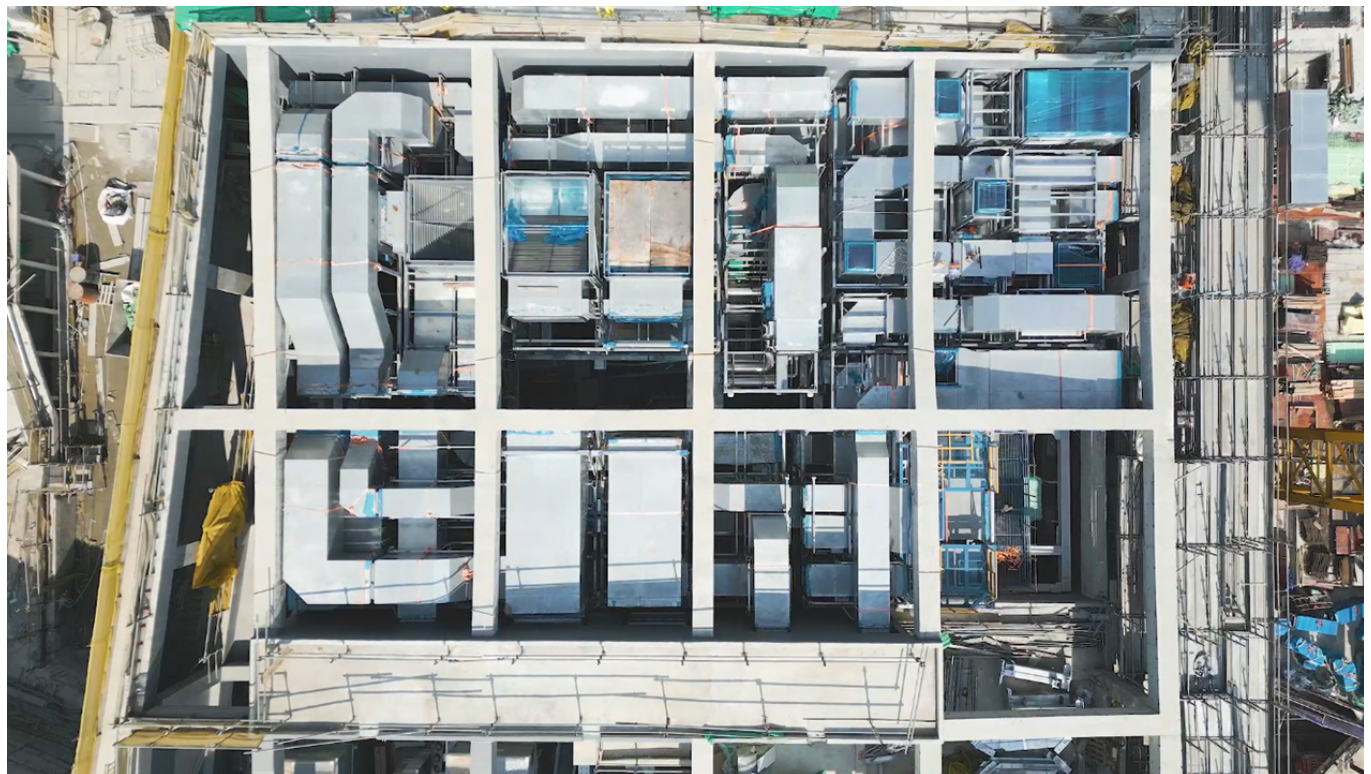
MiMEP units are lowered onto a series of frames and bolted in place to form an entire plant room system
